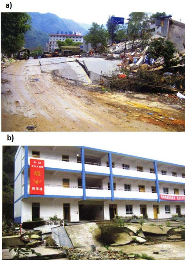
**Fig. 1** Reverse fault rupture examples during the 2008 Wenchuan earthquake in China (a) The road offset vertically by 2m and buildings to the right of the road collapsed, b) The yard of Bailu middle school was offset vertically by 2 m and the building are largely undamaged . [photos adapted from reference 3]
