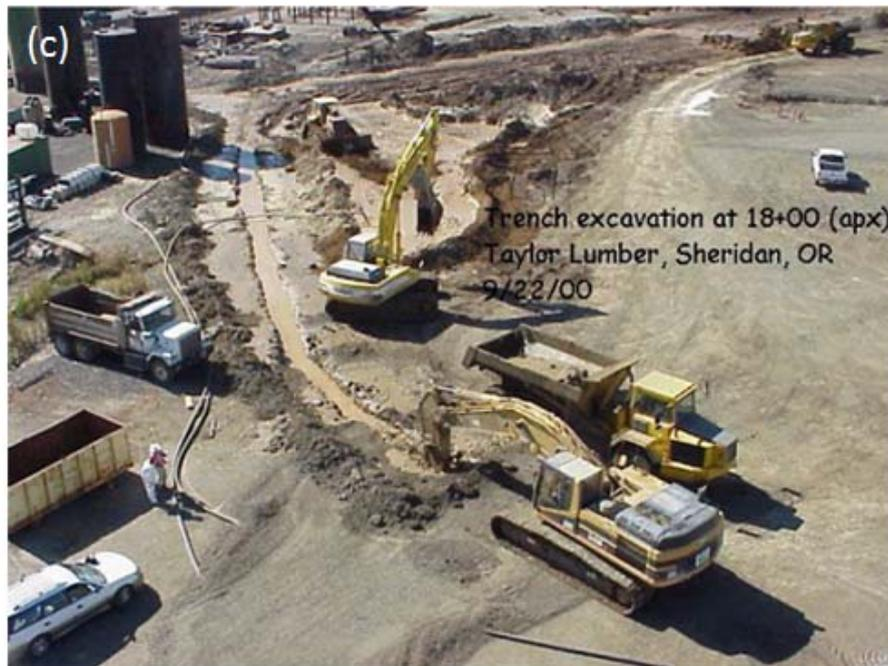
**Fig. 4** The view of construction of soil bentonite soil bentonite wall a) Excavation of trench in the soil under presence of bentonite b) mixing the soil with bentonite and pouring again in the trench c) top view of excavated soil bentonite wall [photos adapted from reference 20]
