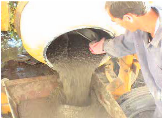
Fig. 1. Mixing of SCLWC
