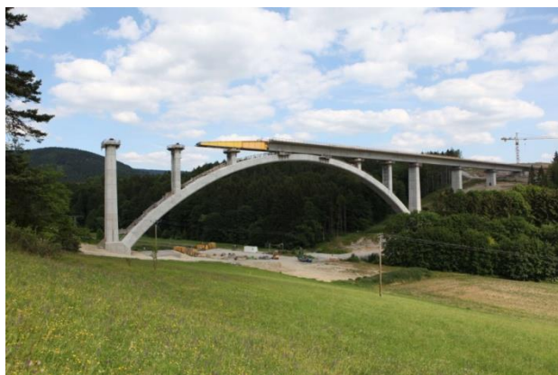
Fig. 1 Incremental bridge launching [1]
